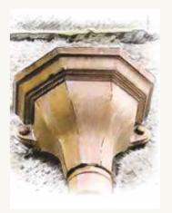
Rainwater goods includes, rhones (gutters), hoppers, brackets downpipes and shoes at the foot. Cast iron was traditionally used because of its durability. If properly maintained these elements have a long life.
