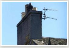
Chimney stacks (called 'stalks'), are the parts of the building most vulnerable for weathering, being exposed on all faces.
