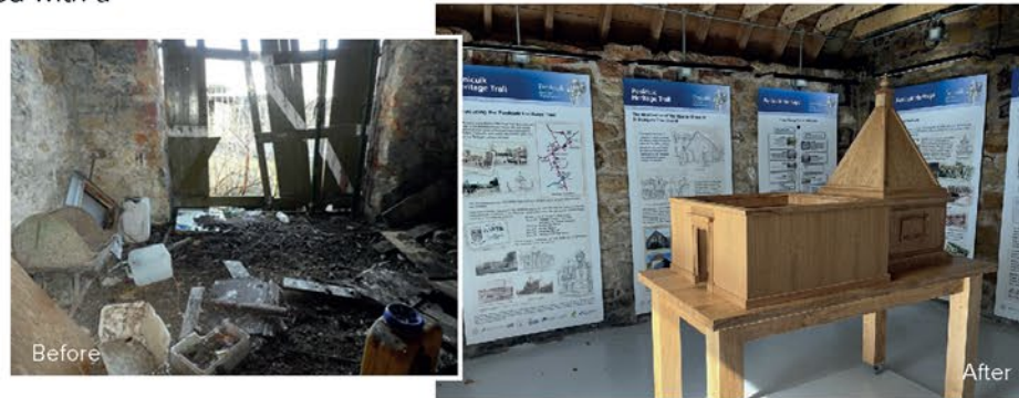
Exterior (top) and interior (above) of the Hearse House
